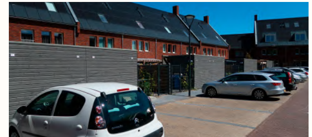
Well-detailed rear parking court, Rotterdam
