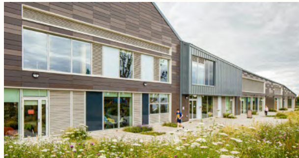
Springfield Community Campus. Credit Simon Doling and Alec French Architects
