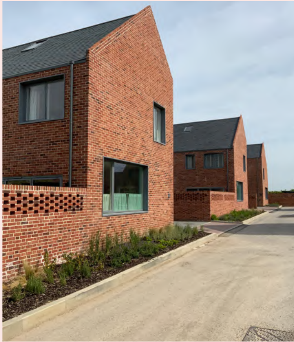
Side gables include large windows to habitable rooms. Boundary walls include perforated brickwork. The Tannery, Holt.
