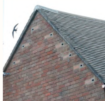
'Universal bricks' integrated within the building's fabric
