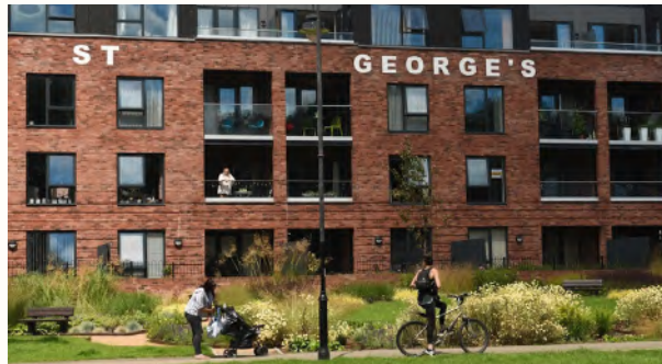
St Georges Works, Trowbridge
