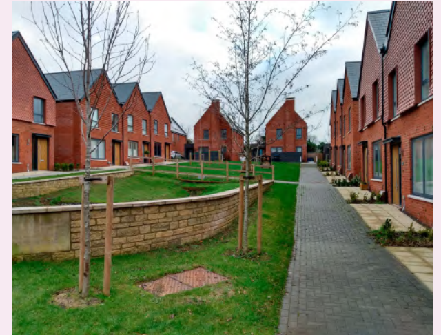
Distinctive gables, tile hanging and chimney stacks, Former Westbury Hospital.
