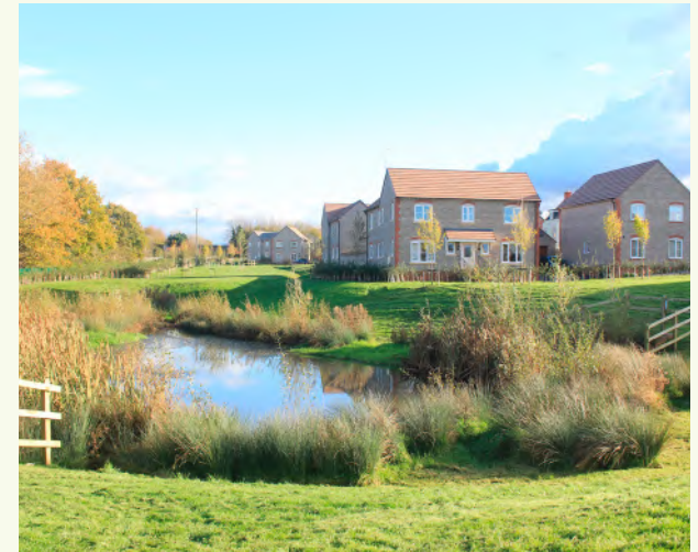
SuDS designed as a natural pond with accessible, split level banks, Ridgeway Farm, Swindon
