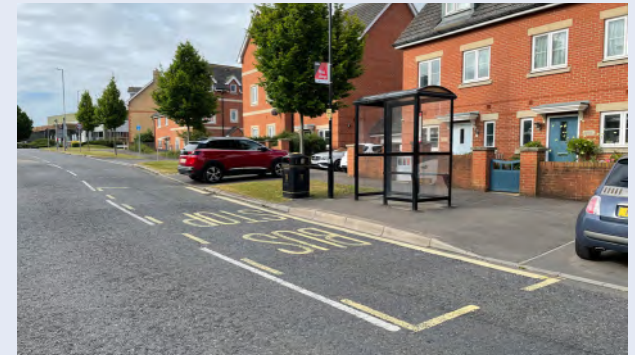
Public realm around bus routes will have additional design requirements, Old Sarum, Salisbury
